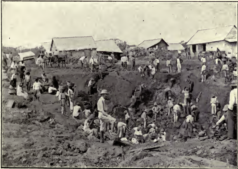
PLATE 19.—Village of La Brea, Trinidad. This is built on pitch, which is shown being dug out by negro workmen.
